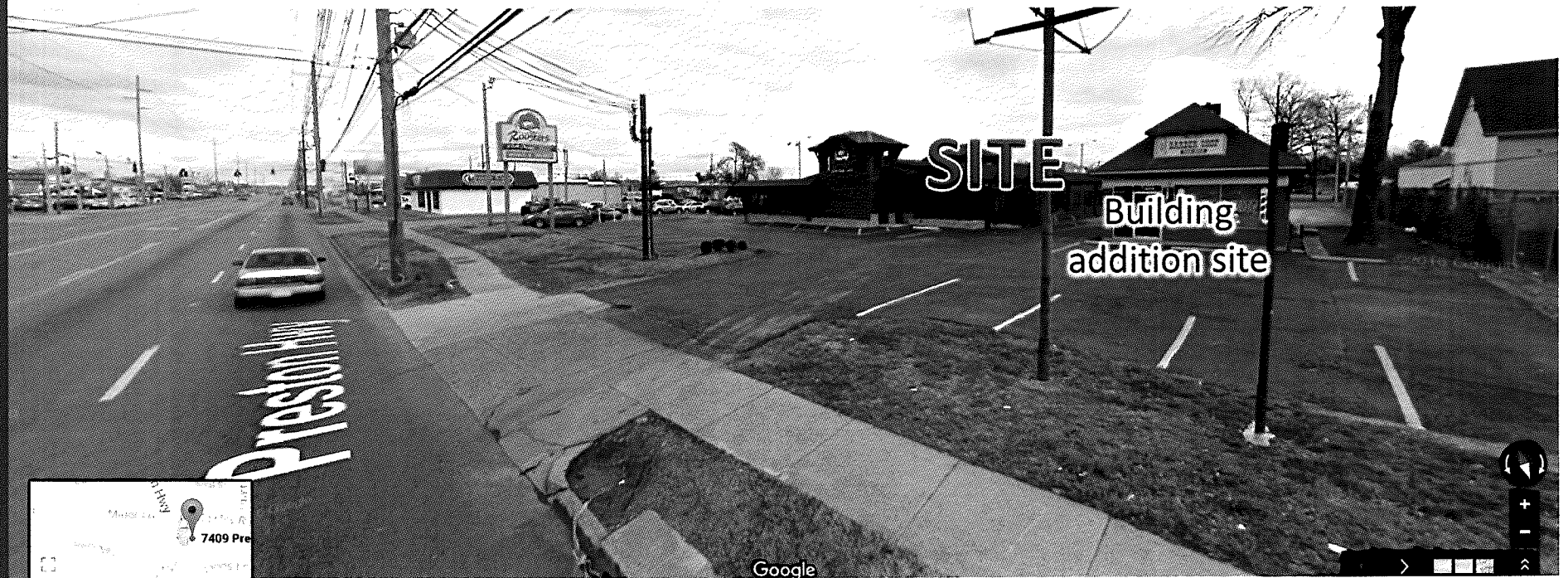
View of site from Preston Highway looking northwardly towards McCawley Road.
