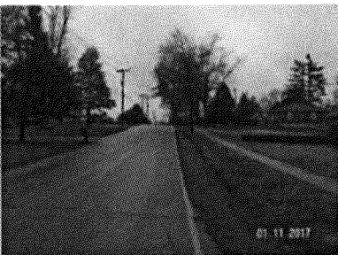
SB Fern Creek 600 ft From Beulah Church Road
