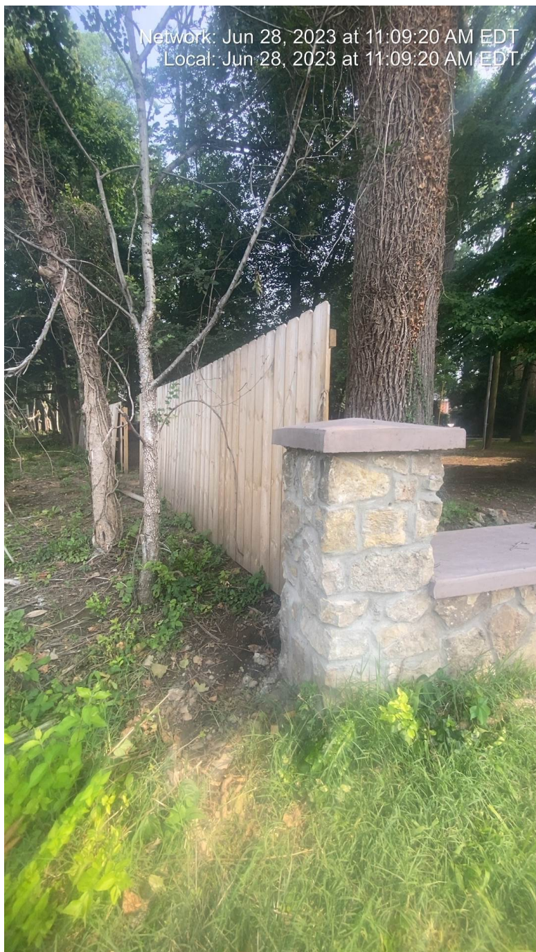
Fence in the side yard.
