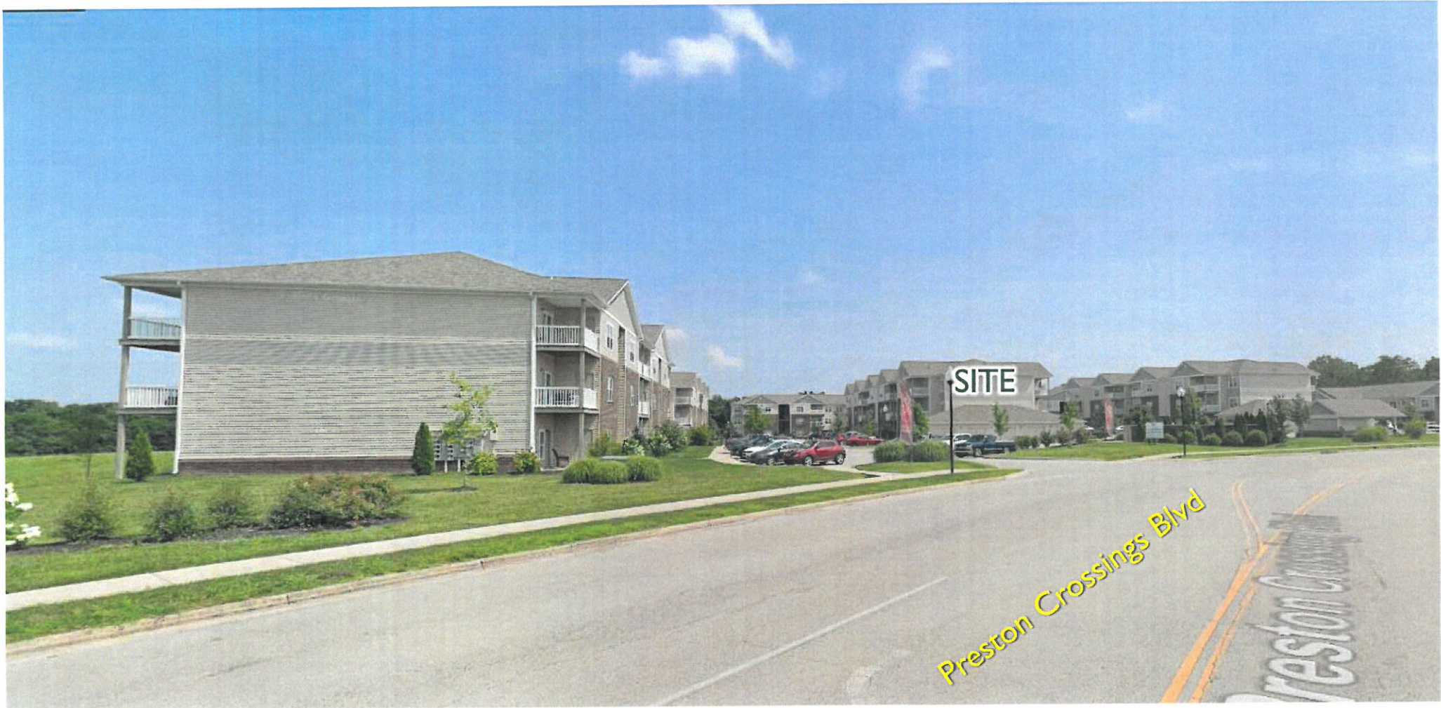
View of site from Preston Crossings Blvd.
