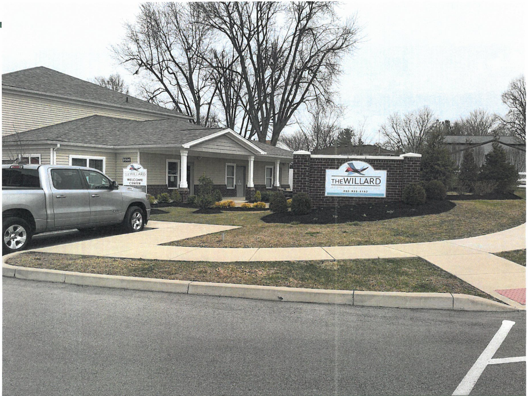
Entrance and Welcome Center/office
