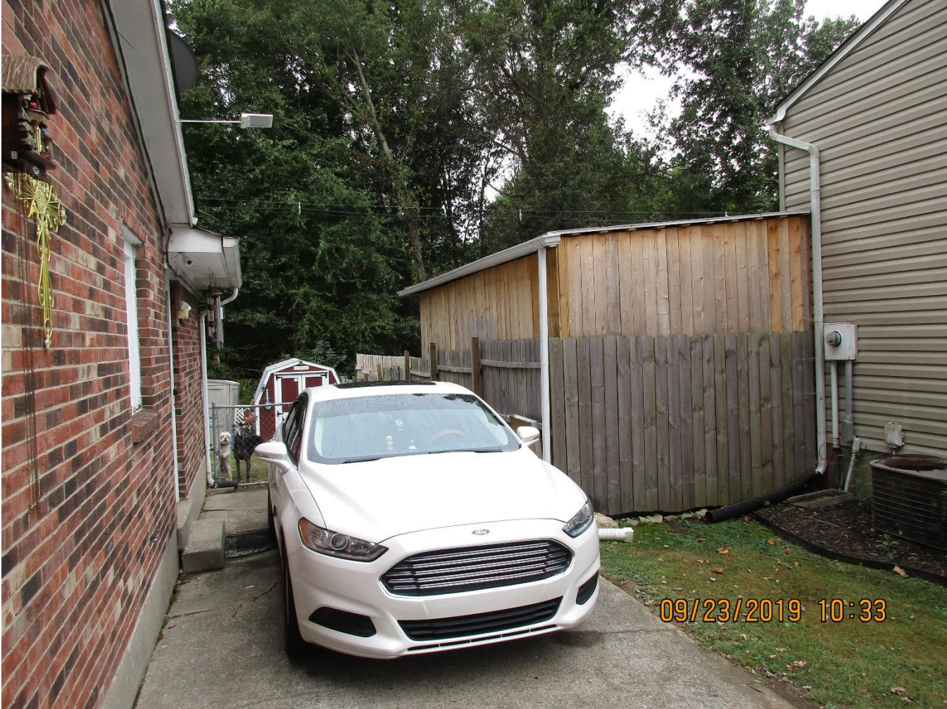
Deck and fence.
