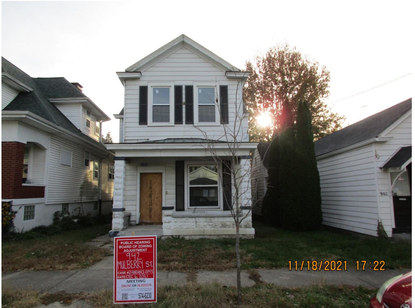
Front of subject property.
