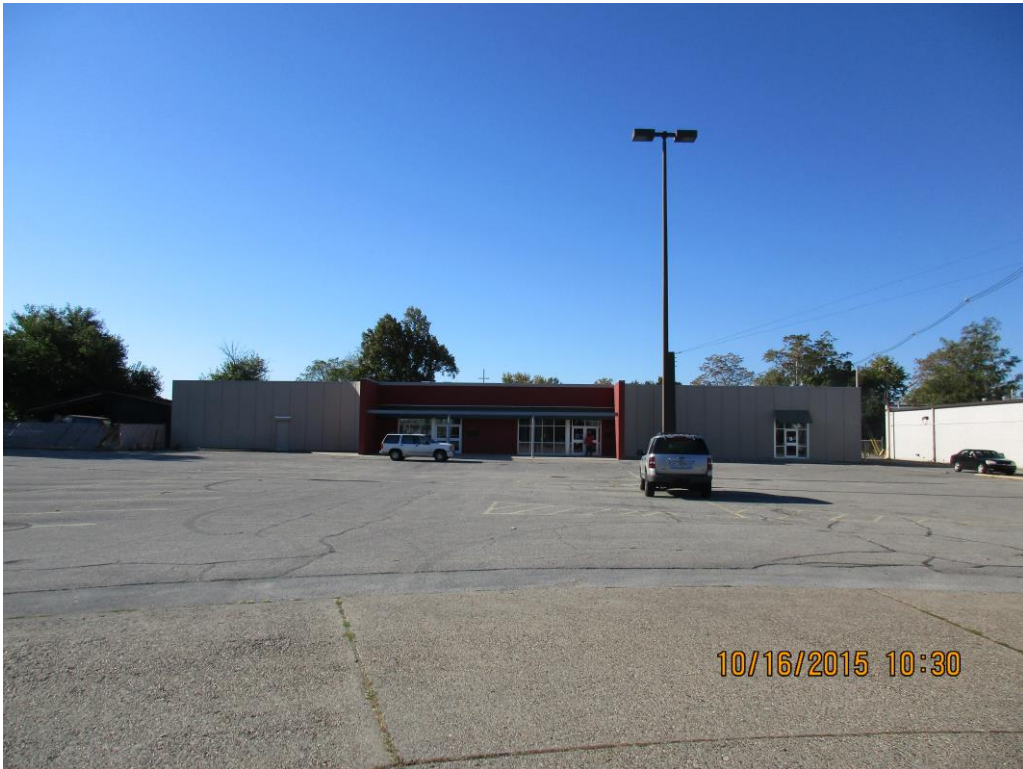
Existing parking in front of the Building
