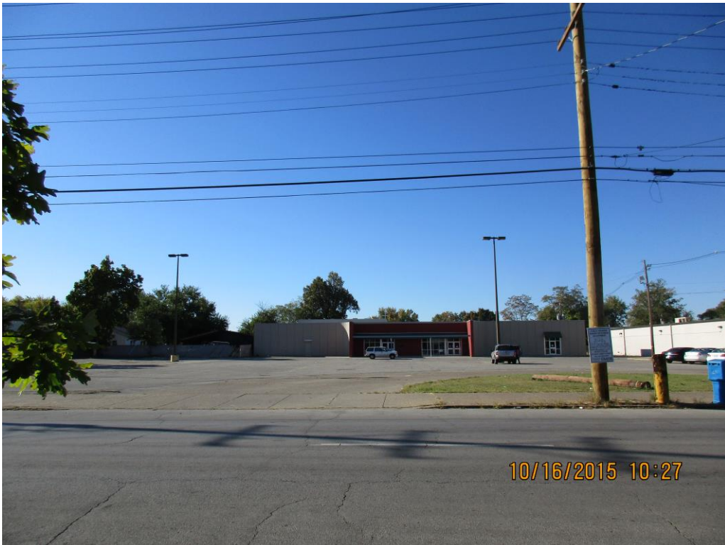
Existing parking lot and front of building
