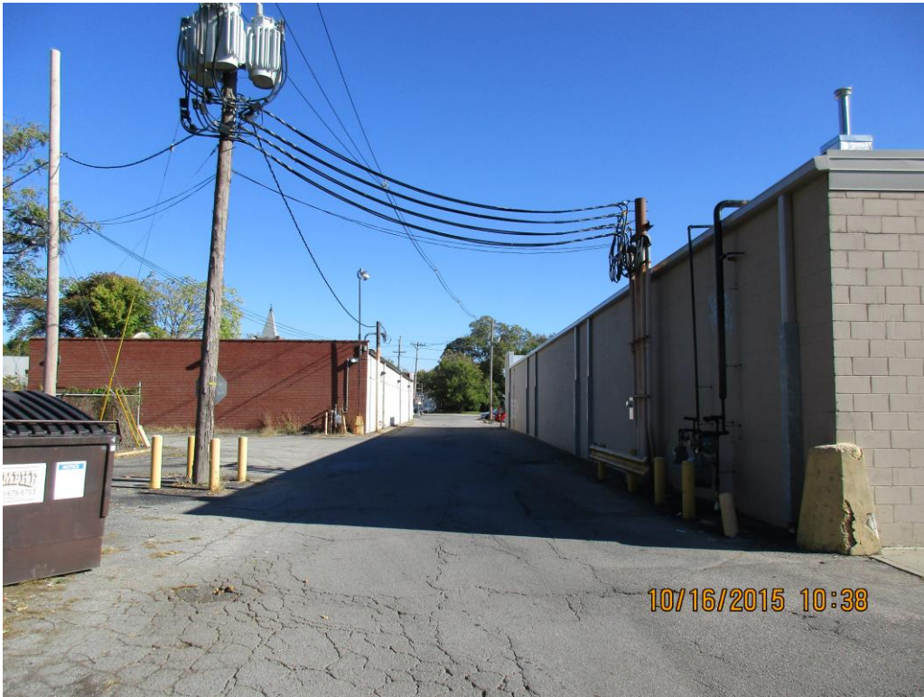
Western Perimeter looking north toward Portland Ave
