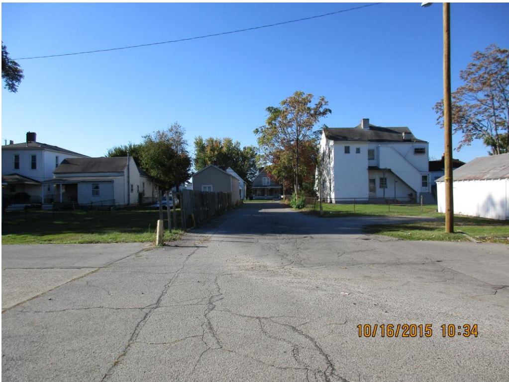
Existing access to Bank Street looking south. Location of the side yard variances.
