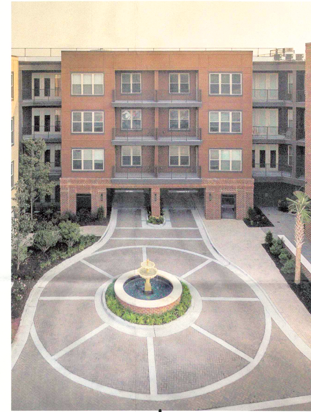
PARKING ENTRANCE and BALCONY DETAIL
