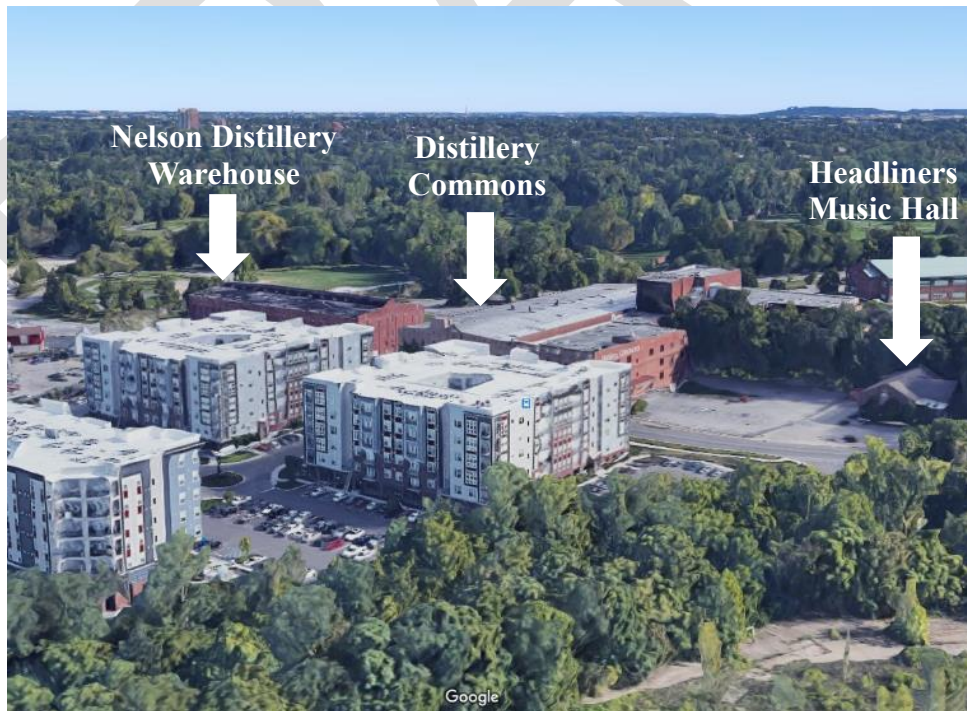
Google Photo showing the locations of the Nelson Distillery Warehouse and other extant buildings.
