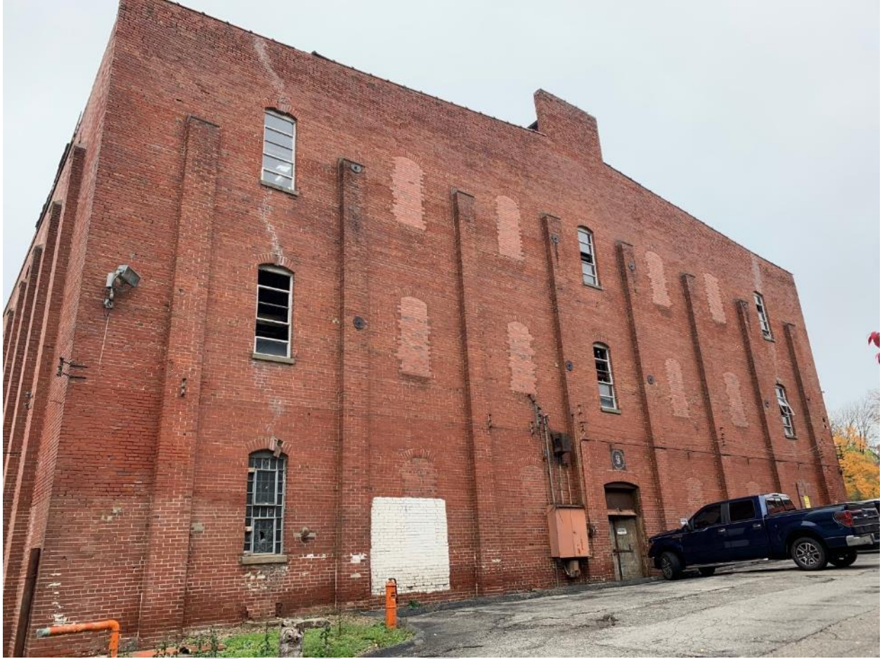
West Elevation (Staff Photo October 2020)
