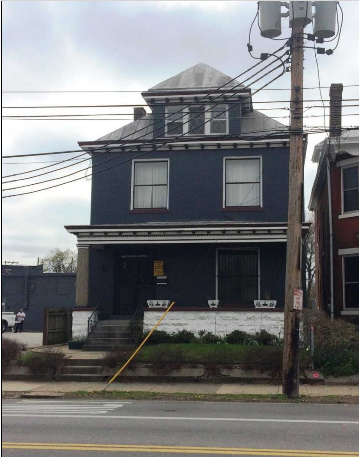
Image 10. North, front, elevation of 1240 E. Broadway.
