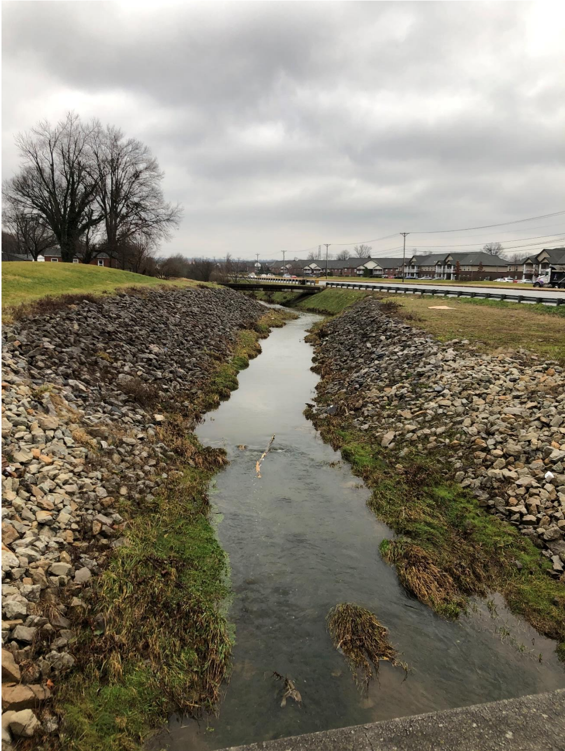
Location of Spring Ditch facing east.
