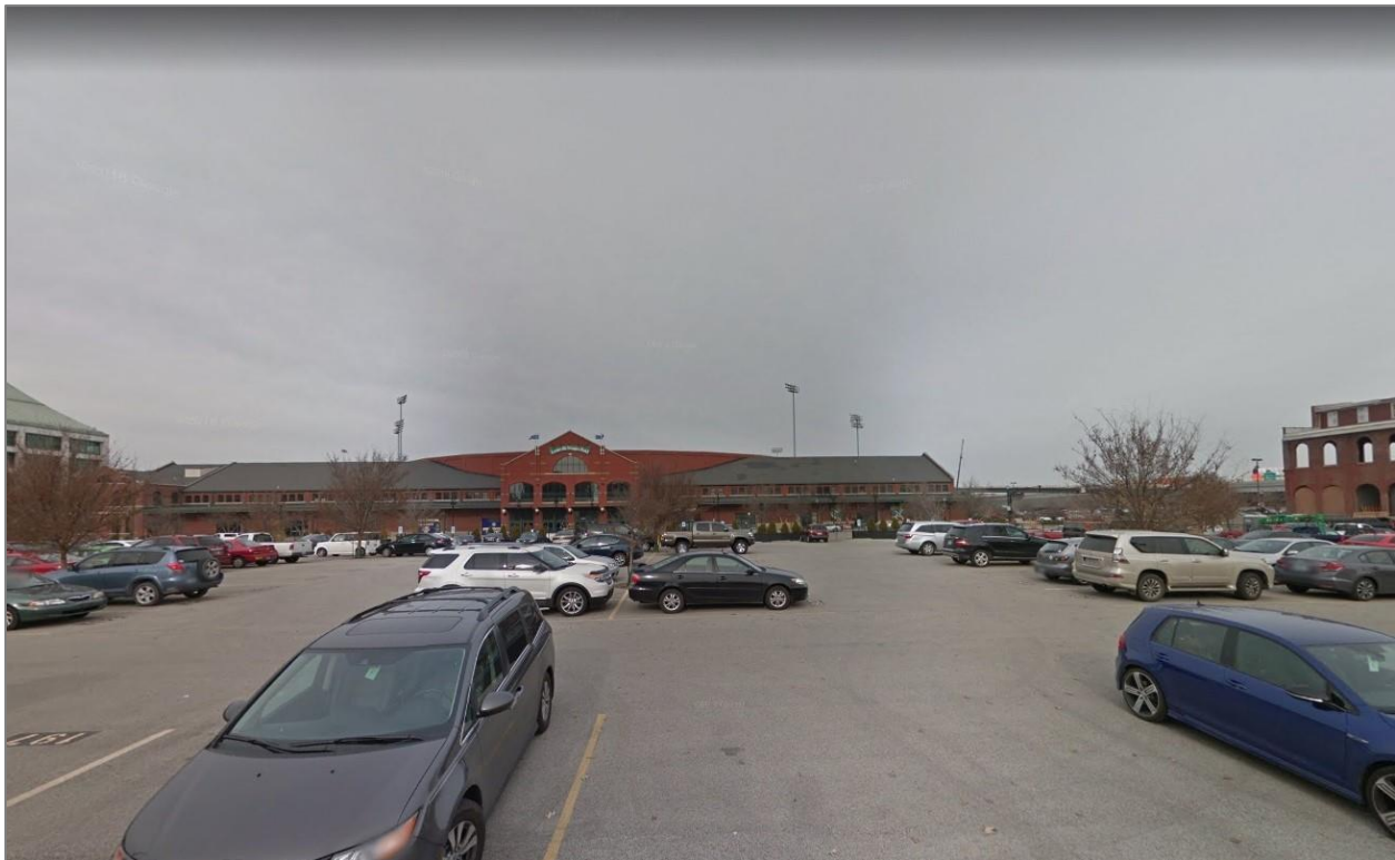
418 E Main Property from the Alley Google December 2015
