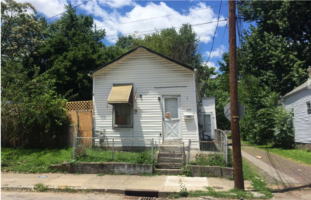
Front view-314 N. 21 st Street (Applicant's property)
