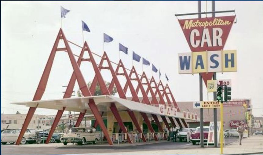
Metropolitan Car Wash, Los Angeles Ca.
