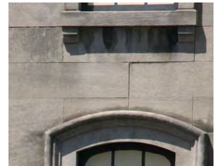
Fig 23: 813, cracked stone & mortar
