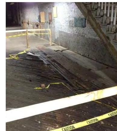
Fig 14: 811, 1 st floor apparent water and termite damage
