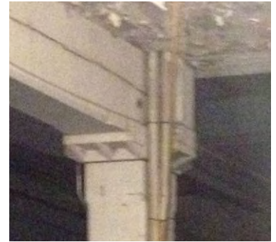
Fig 11: Cast-iron column connection
