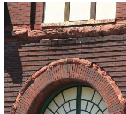
Fig 19: Deteriorated sandstone elements and bowing brick
