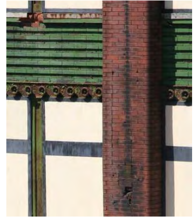
Fig 20: 815/817, cracked brick & mortar
