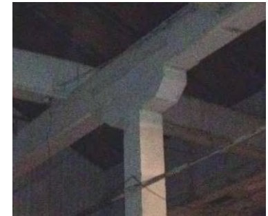
Fig 12 : nailed gravity connection
