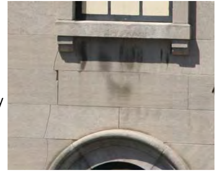
Fig 22: 813, cracked stone & mortar
