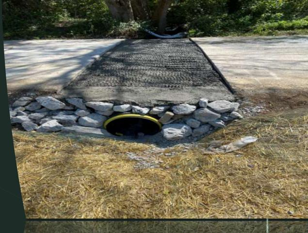
CHEMICAL FIRE DAMAGES RESULTING IN ROAD AND CULVERT REPAIRS — OLD TAYLORSVILLE ROAD
