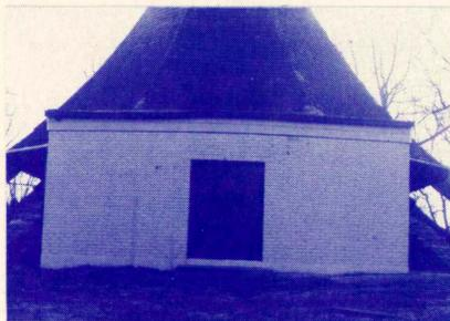
REPLACE GUTTER WITH SEAMLESS ALUMINUM GUTTER AND DOWNSPOUT. PAINT BUILDING, DOORS AND GUTTERS AS SPECIFIED.
