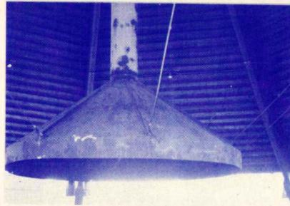
REMOVE/REPLACE HOOD AND LOWER TWO FLUE SECTIONS OR REMOVE ENTIRE HOOD/FLUE ASSEMBLY AS DIRECTED (BID ALTERNATE). TURNBUCKLES TO BE INSTALLED ON SUPPORT RODS.
