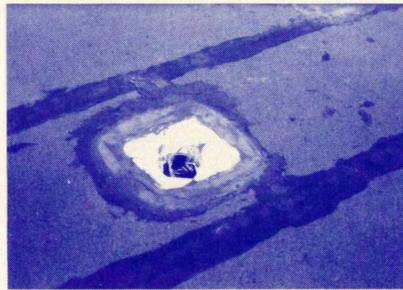
TYPICAL: REPLACE STATIC VENTS ON RESTROOM BUILDING.
