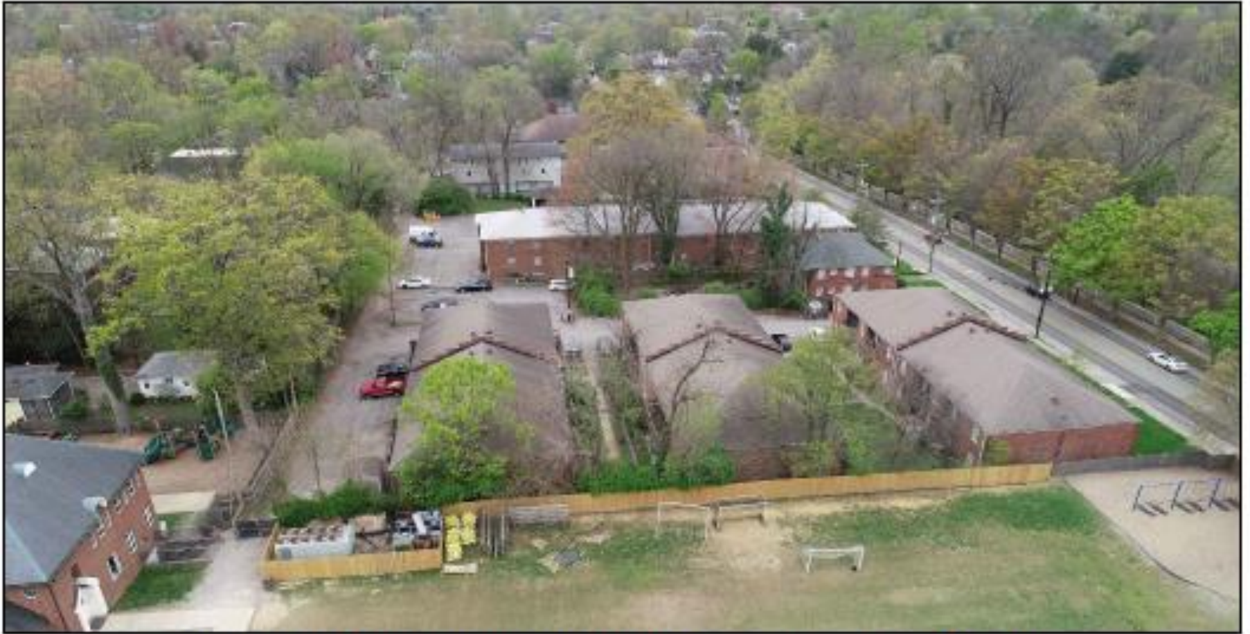
YORKTOWN TO THE NORTHWEST - YORKTOWN APARTMENTS TO BE DEMOLISHED
