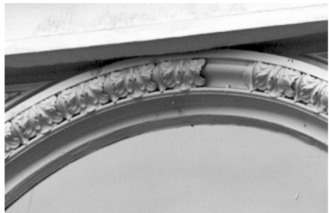
Top left—rust-induced railing deterioration; top right—cast-iron piers; above left—decorative metal lantern; above right—attached foliate cast-iron ornament.
