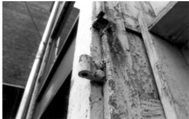
(Middle and Below) In addition to its use as a decorative device, paint serves an important preservative function for some materials. If left exposed to the elements, wood and metal deteriorate rapidly as seen here.
