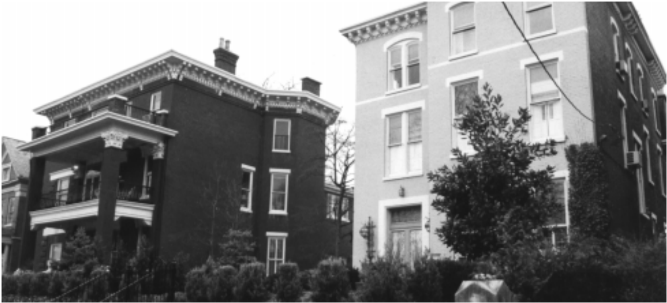
(Above) The color, texture, and shape of masonry and mortar joints contribute to a building's architectural character. Painting masonry, as seen in the example above, significantly alters each of these elements, changing not only a building's facade, but how that building relates to neighboring structures.
