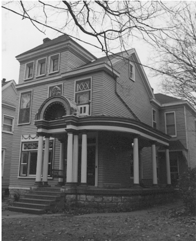
Porches help to personalize many of Louisville's residences and apartment buildings. Some, such as the one above, are flamboyant, while others are more reserved.
