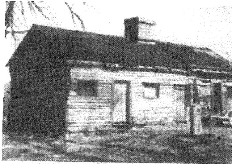
**Figure 4. Original double pen log cabin with central chimney.**
