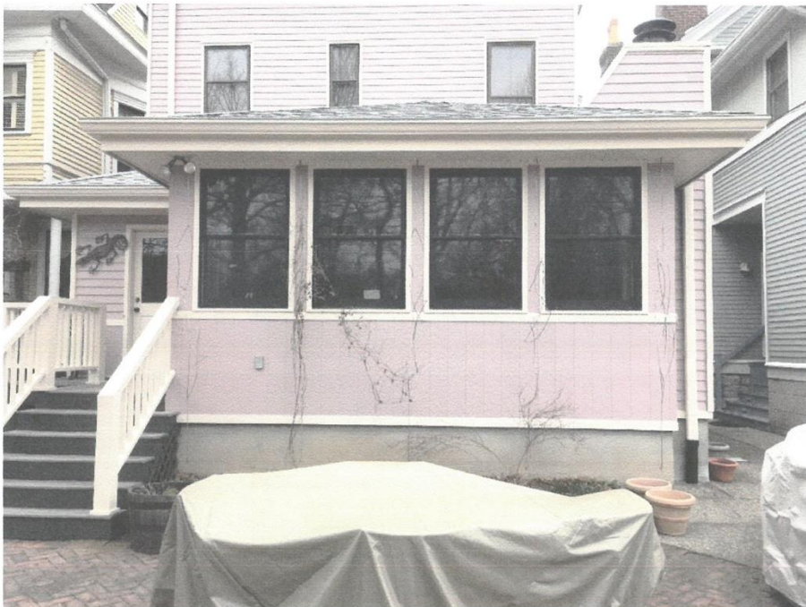
View of rear of addition. Two center window will be replaced with a French sliding door.
