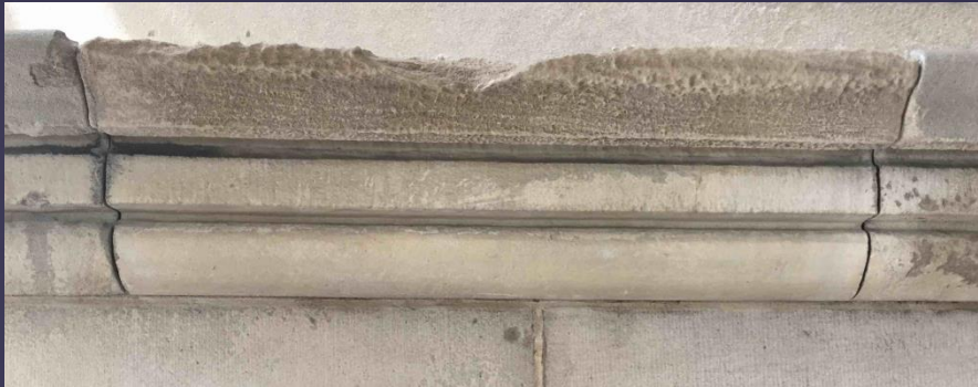
Existing Limestone Water Table Before Structural Repairs
