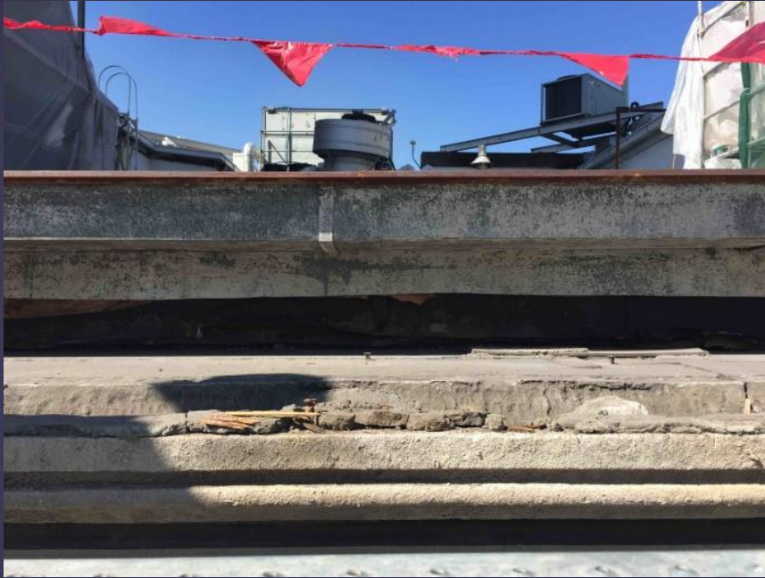
Existing Gutter & Roof Edge Before Structural Repairs
