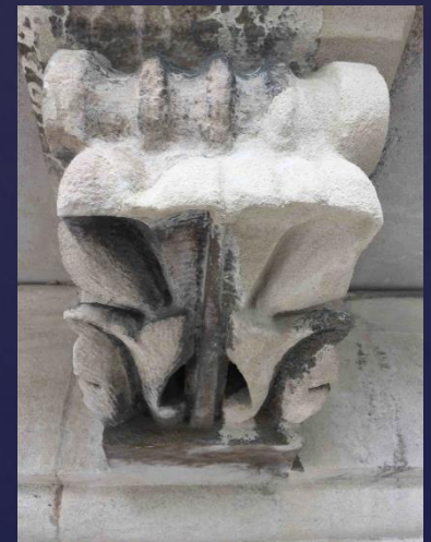
Existing Limestone Bear Claw After Structural Repairs
