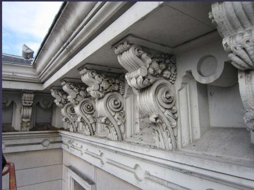
Limestone Corbel Before Cleaning
