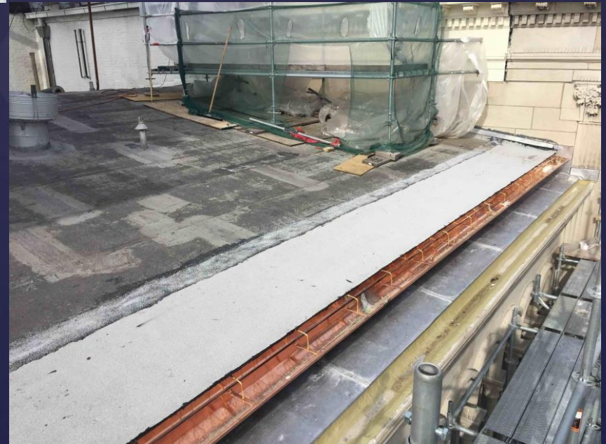
New Copper Gutter & Roof Edge After Structural Repairs
