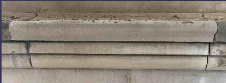
Existing Limestone Water Table After Structural Repairs
