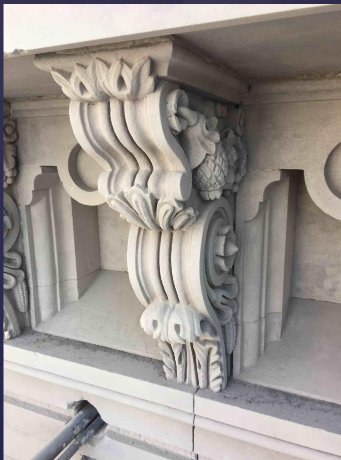
Limestone Corbel After Cleaning
