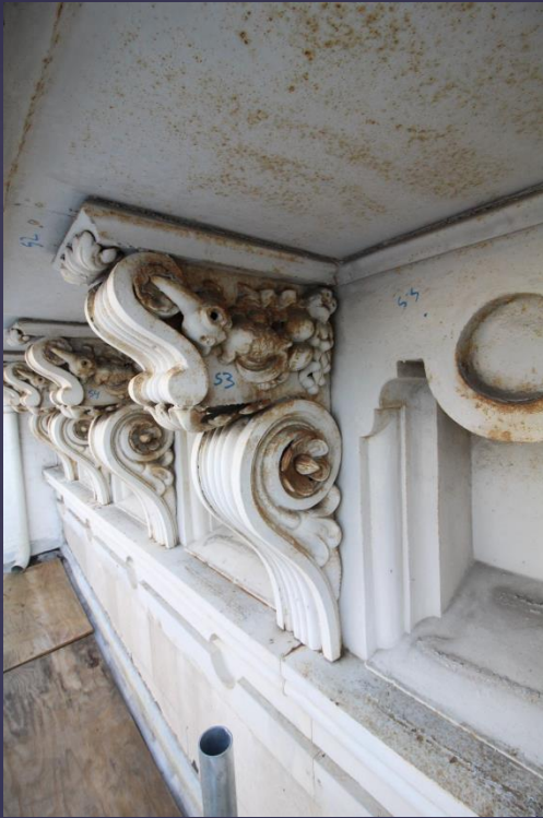
Cast Iron Corbels Before Restoration
