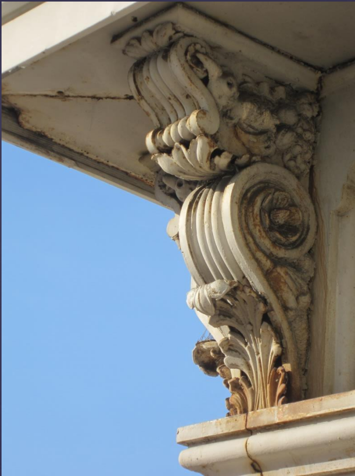
Cast Iron Corbel Before Restoration
