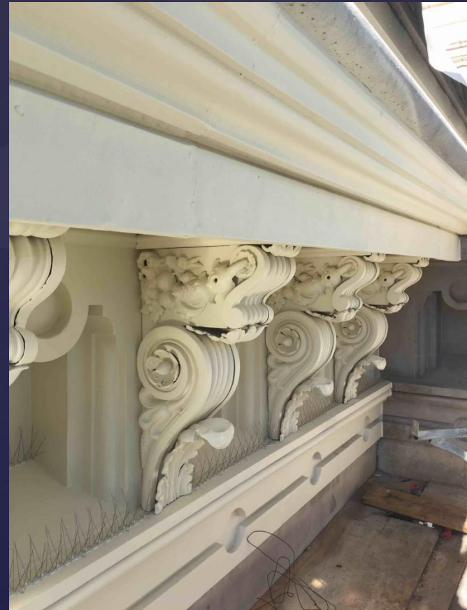
Cast Iron Corbels After Restoration
