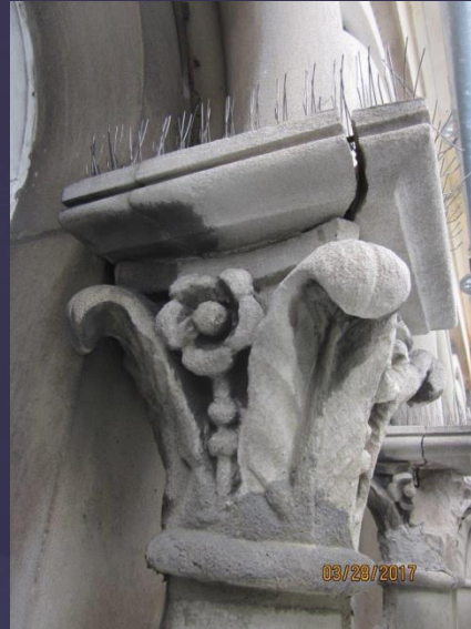
Examples of Typical Stone Column Capitals Before Replacement
