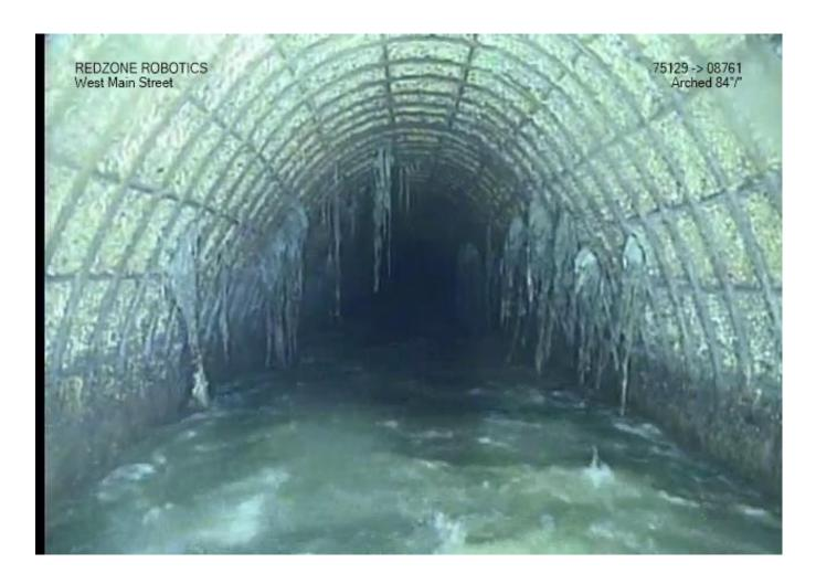
Video and laser inspection show concrete worn away and exposed rebar due to corrosion from sewer gases, particularly between 4<sup>th</sup> and 7<sup>th</sup> streets along West Main St.
