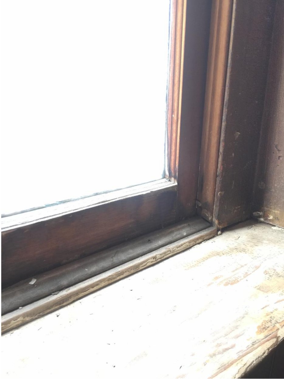
West elevation window #5- class 3-4
