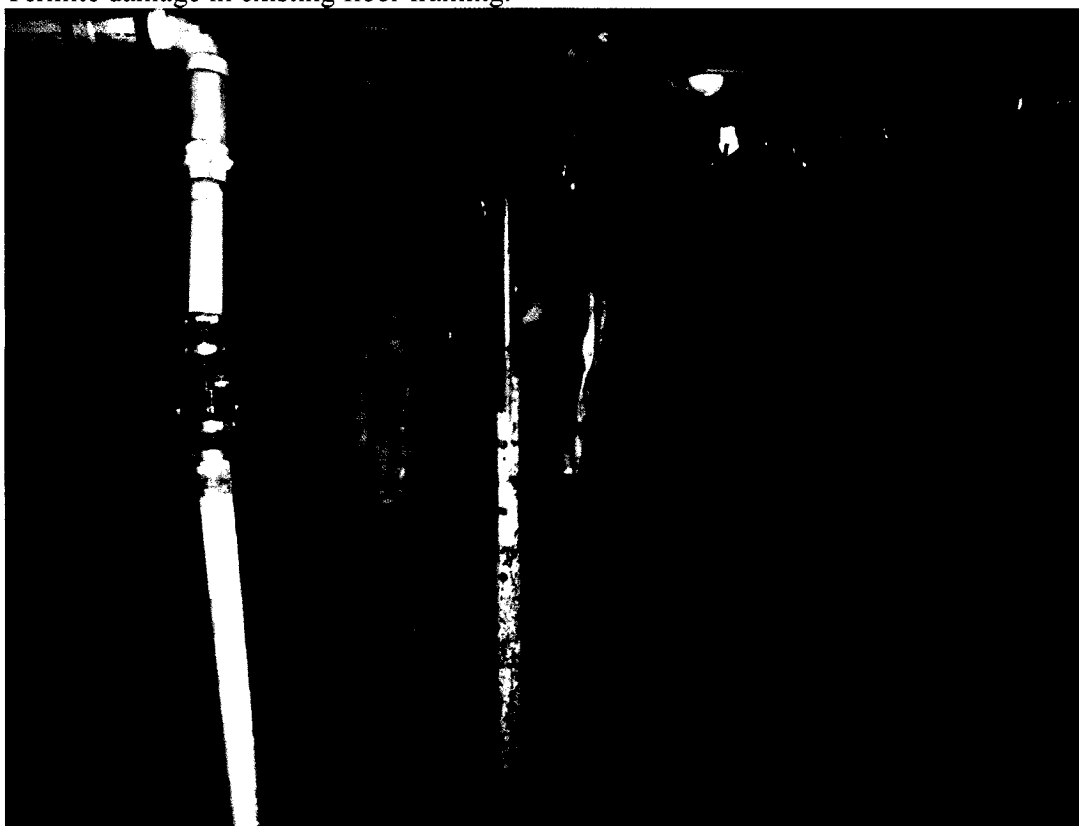
Steel posts placed to shore the existing floor framing.
