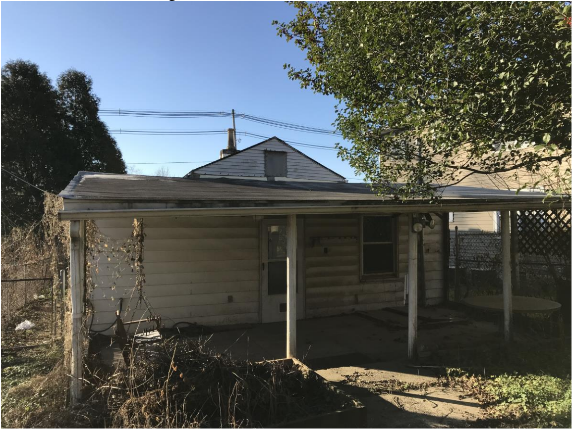
Rear Elevation of Building
