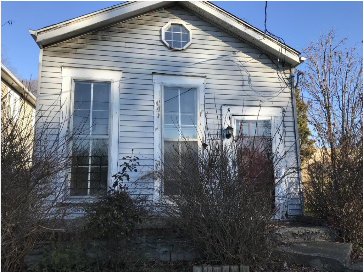
Front Elevation of Building
