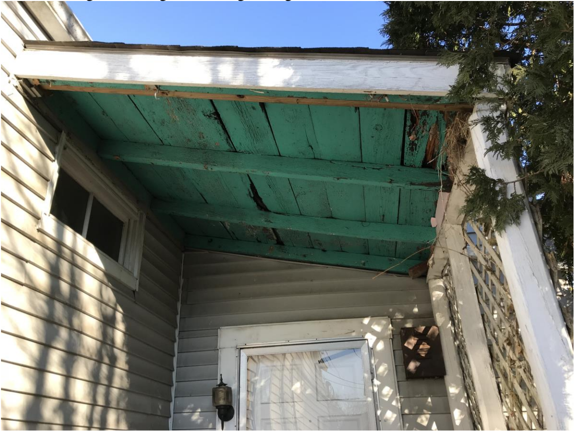
Side door porch roof framing.
