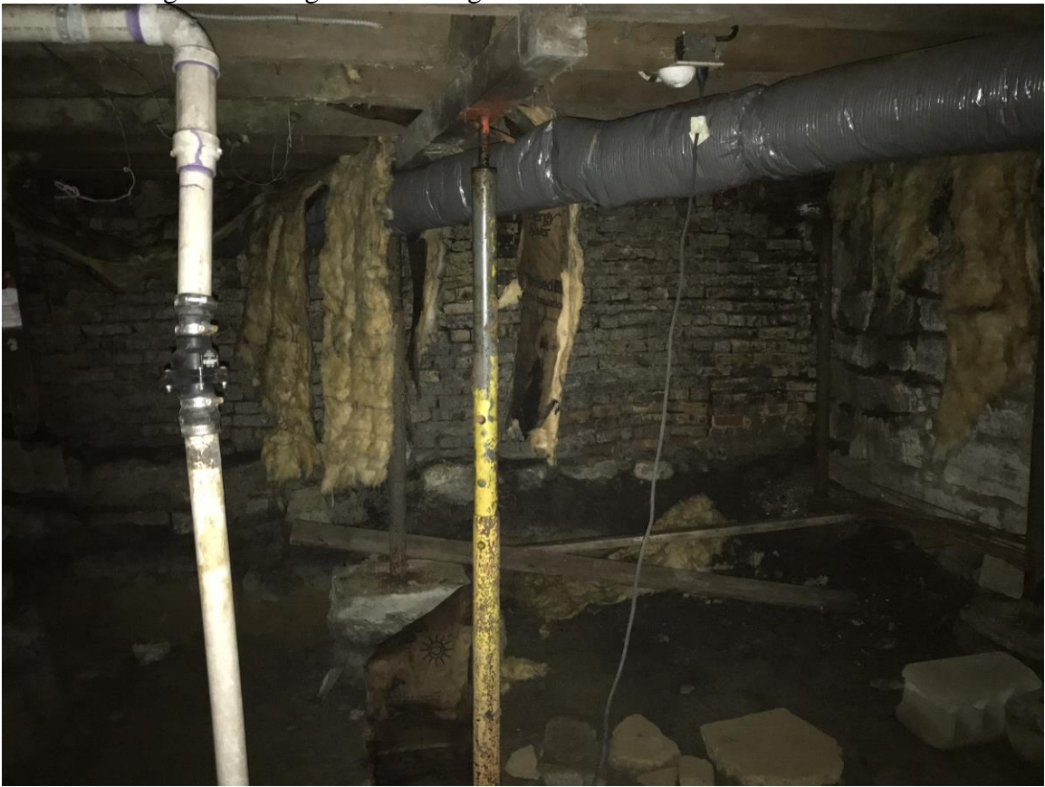
Steel posts placed to shore the existing floor framing.
