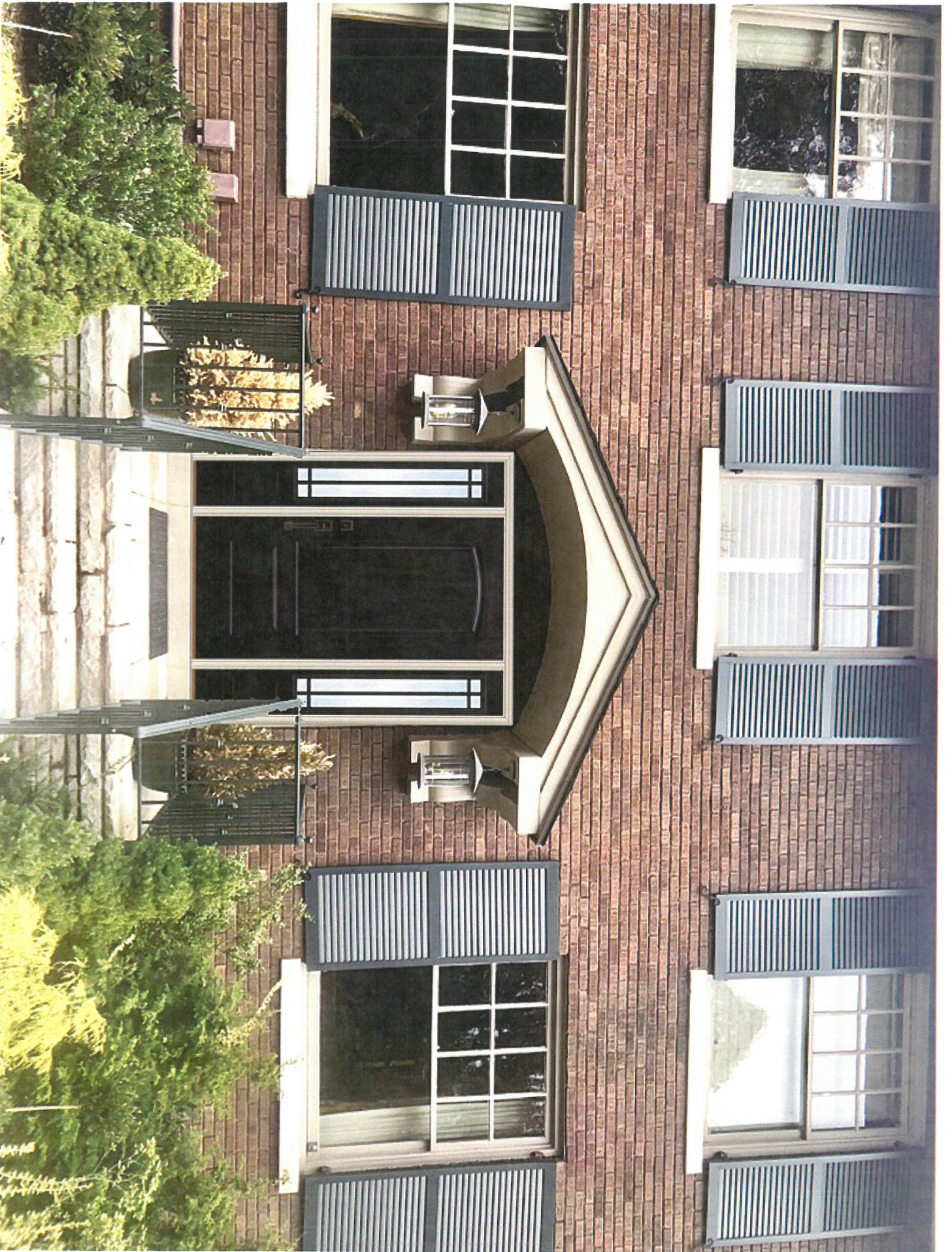
PHOTOSHOP OF NEW DOOR. SIDE LIGHTS WILL BE SLIGHTLY WIDER AND FLUSH AT BOTTOM WITH A MAIL SLOT.
