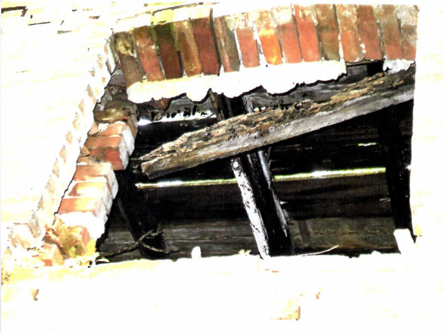
Deteriorated Window
