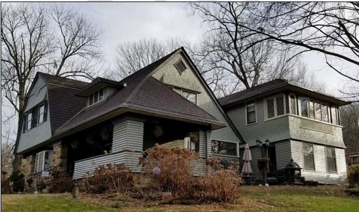
Figure 29. North and west elevations, looking southeast. The second floor sleeping porch enclosed with windows. A vent was added under the gable.
