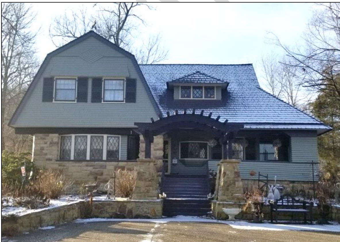
Figure 25. Front façade, or north elevation, looking south. After the fire, the windows in the dormer were converted from two to three and the chimney was not rebuilt.
