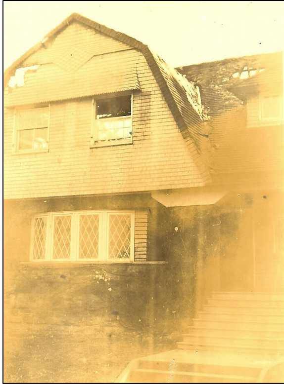
Figure 15. 1930 photograph showing fire damage on the roof and front facade (Courtesy of Stefanie Buzan).
