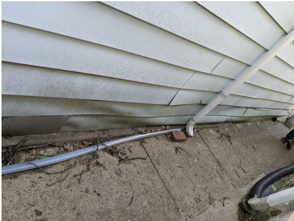
Right side siding buckling
