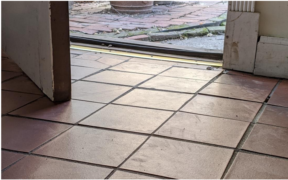
Rear addition floor buckling; interferes with door operation
