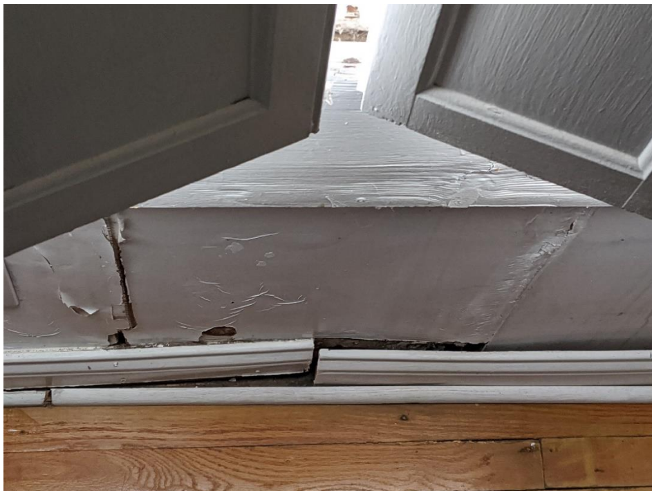
Interior wall buckling roughly halfway along right side
