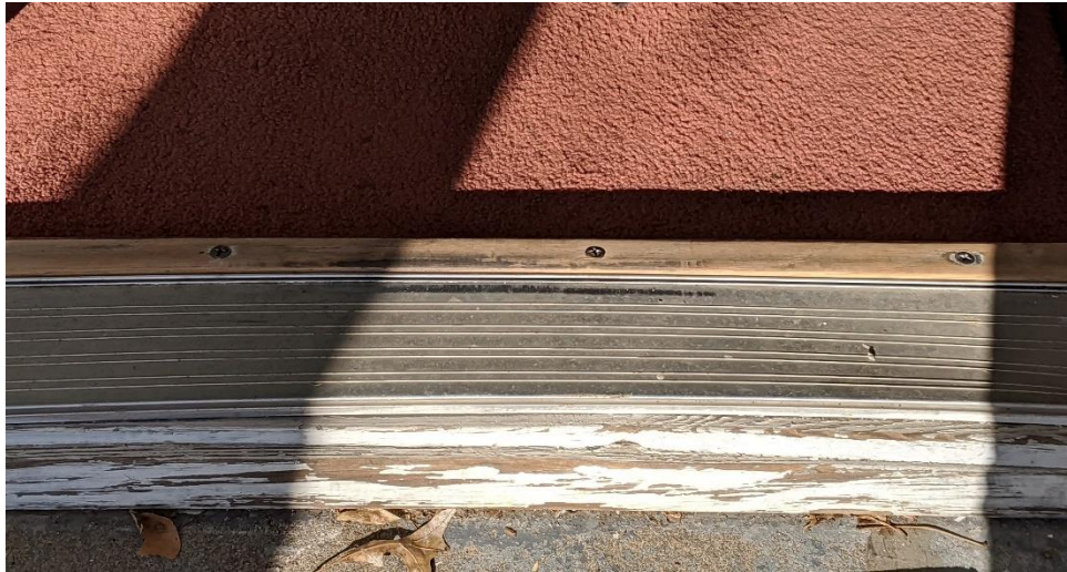
Severely bowed front door threshold
