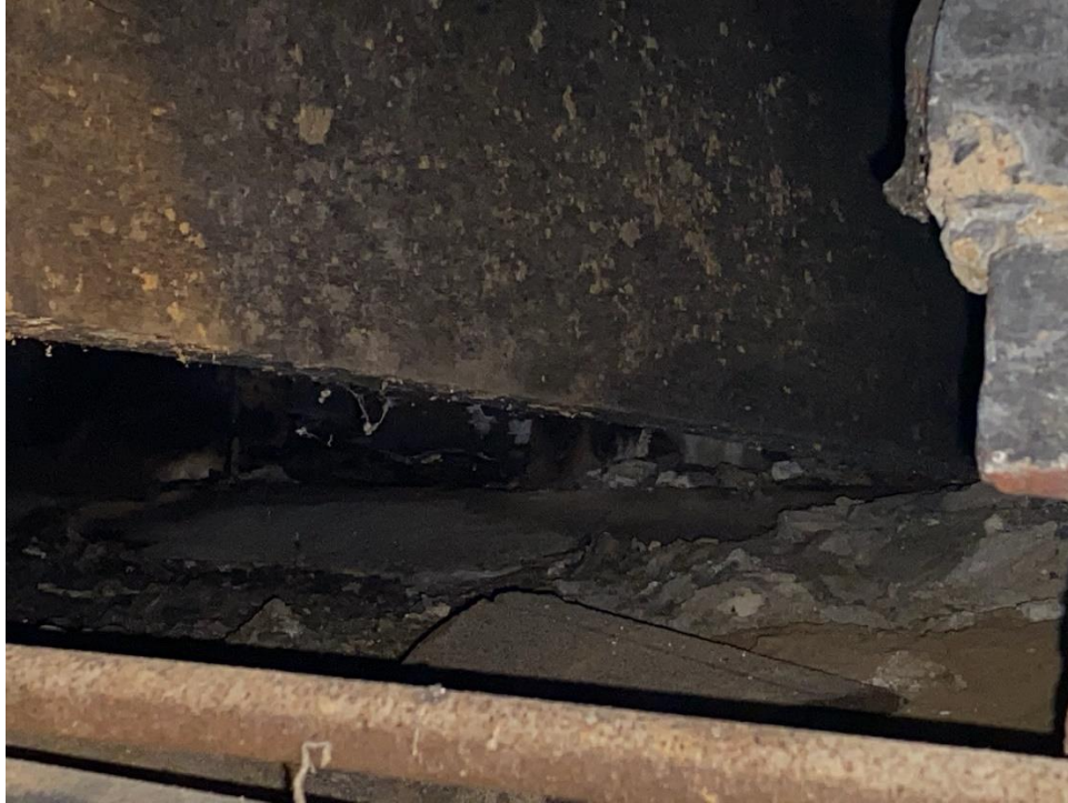
Right front side of home, floor joist sitting on dirt, cedar foundation posts not visible
