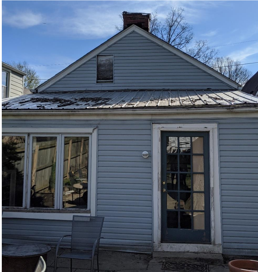
Rear addition with uneven foundation/pavement, door no longer square
