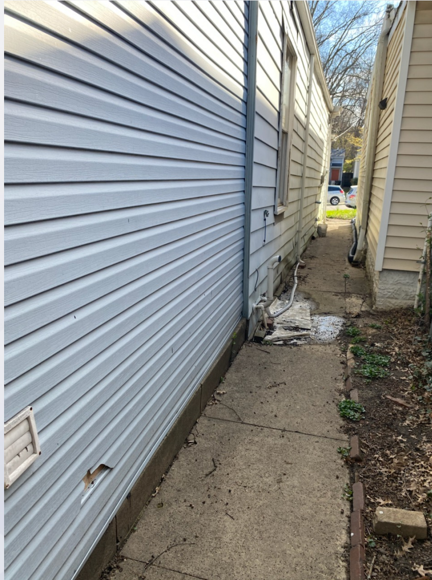
South side wall is wavy and bulging
