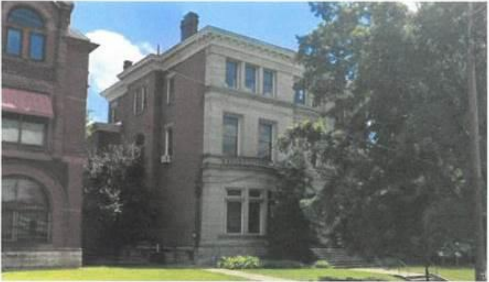
The front of 1215 S. 3rd Street, from just north of the building facing southeast.
