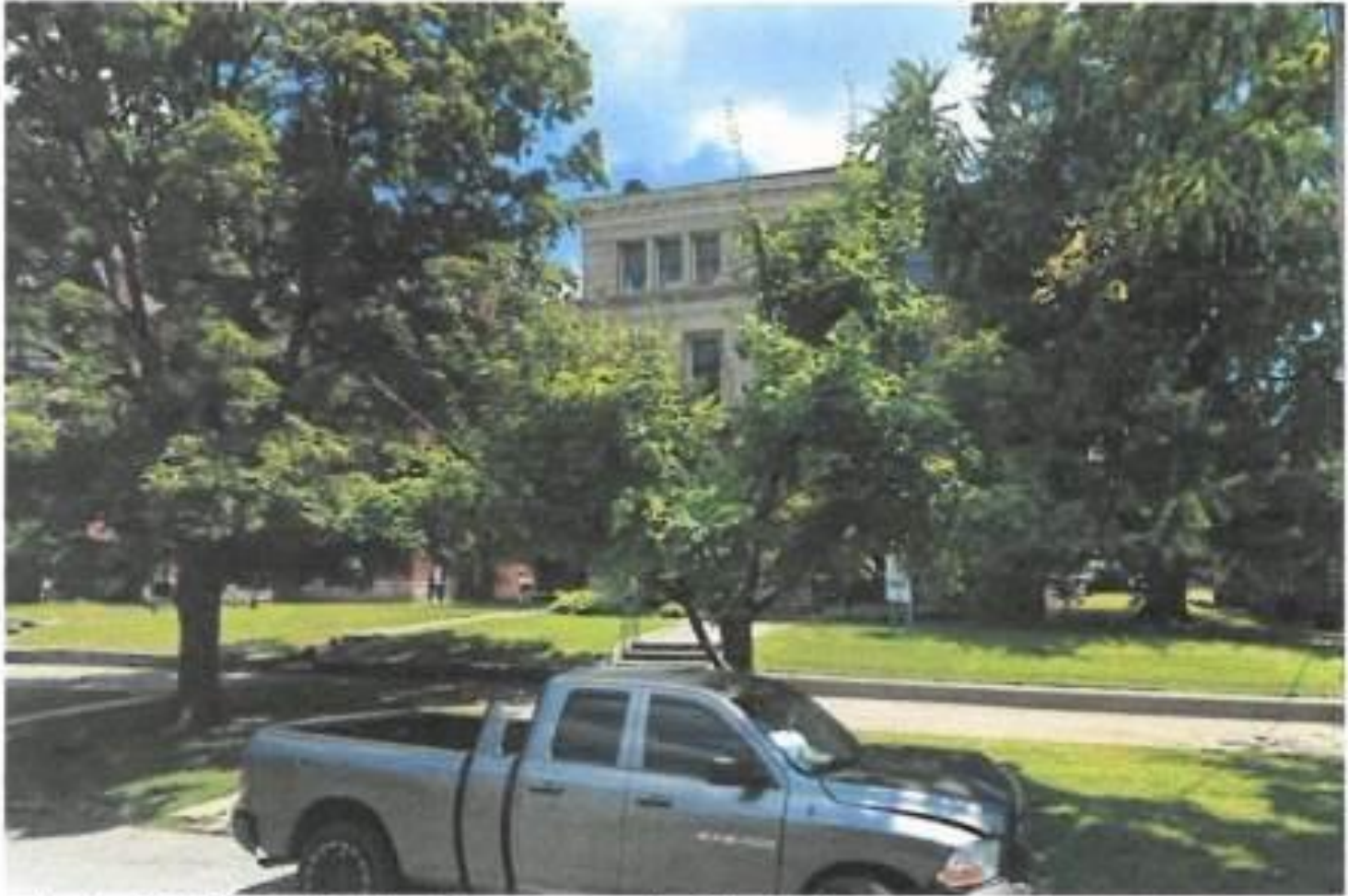
The front of 1215 S. 3rd Street, from just south of the building facing northeast.
