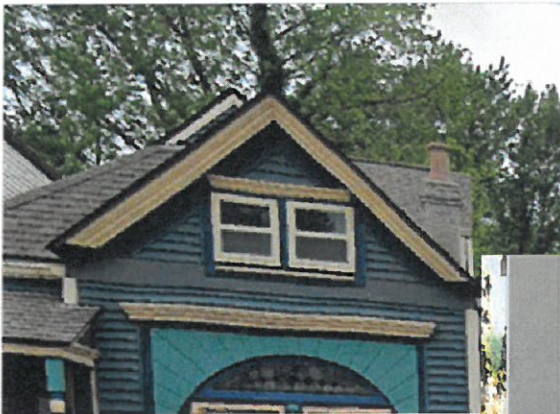
Neighborhood Precedent of Commonly used Gables, Windows and Siding
