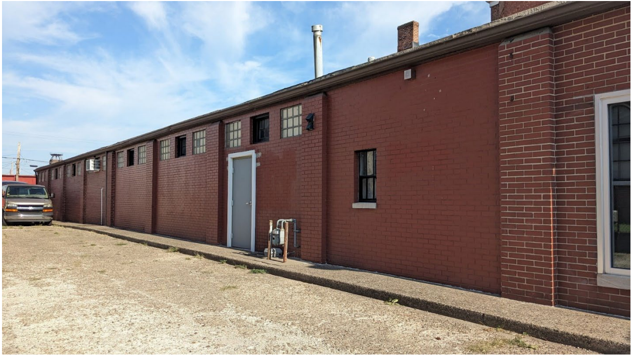
South Side Façade
