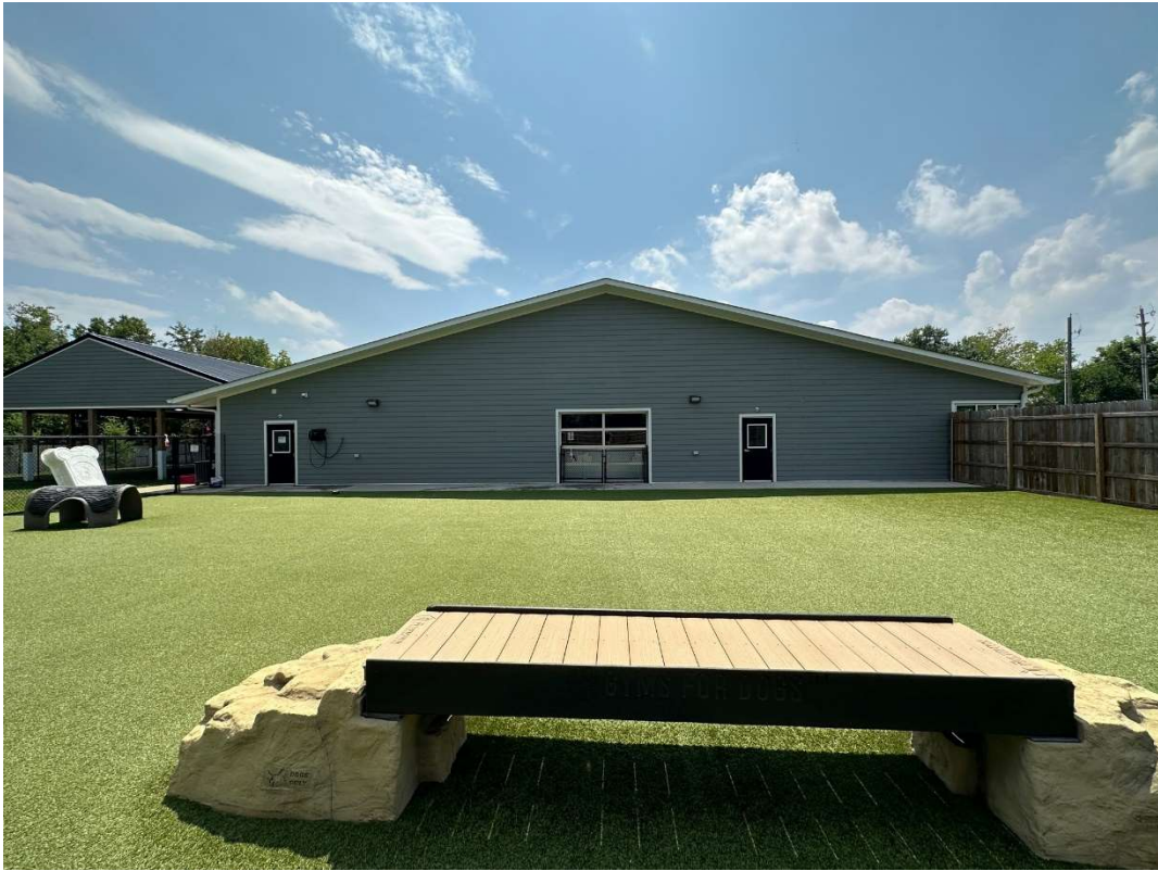
Indoor Park Building – Side View (left)
