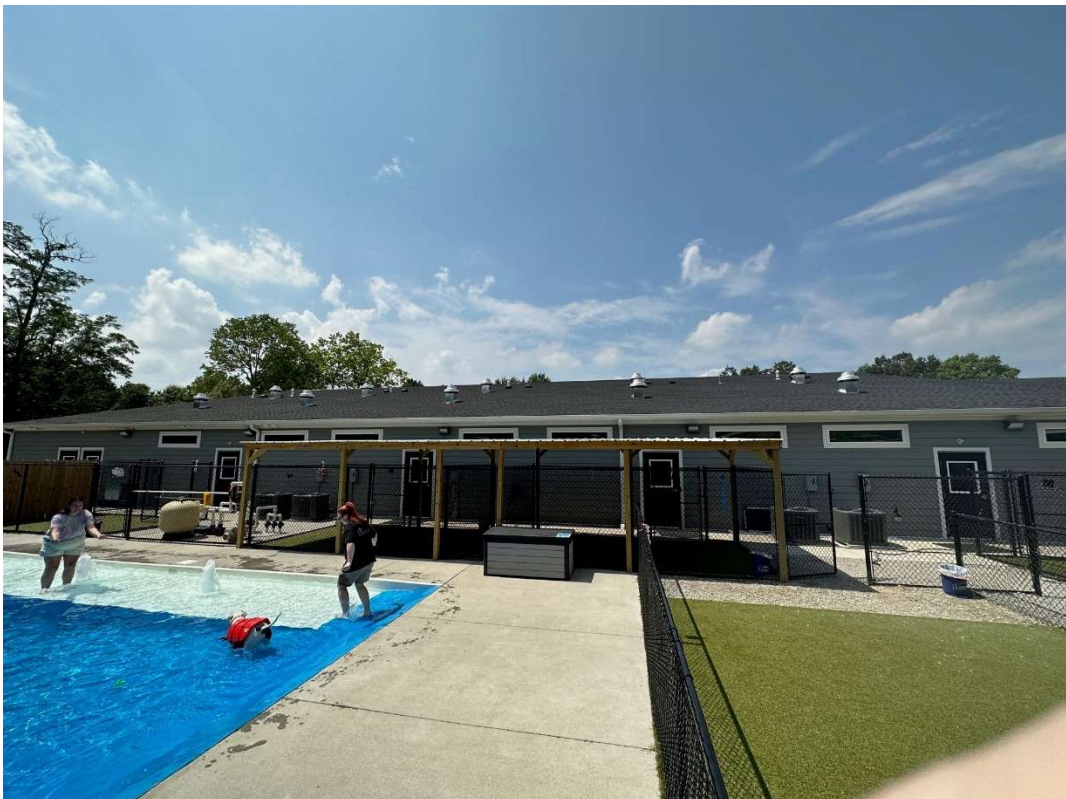
Kennel Building – Rear View
