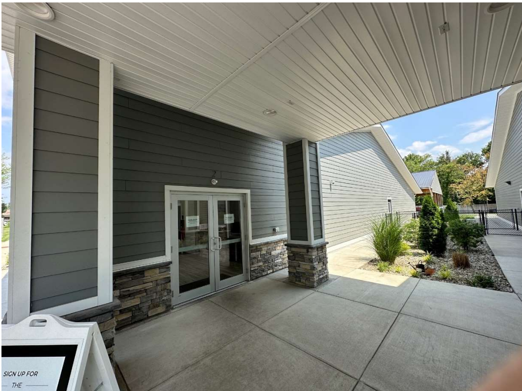
Indoor Park Building – Side View (Right)
