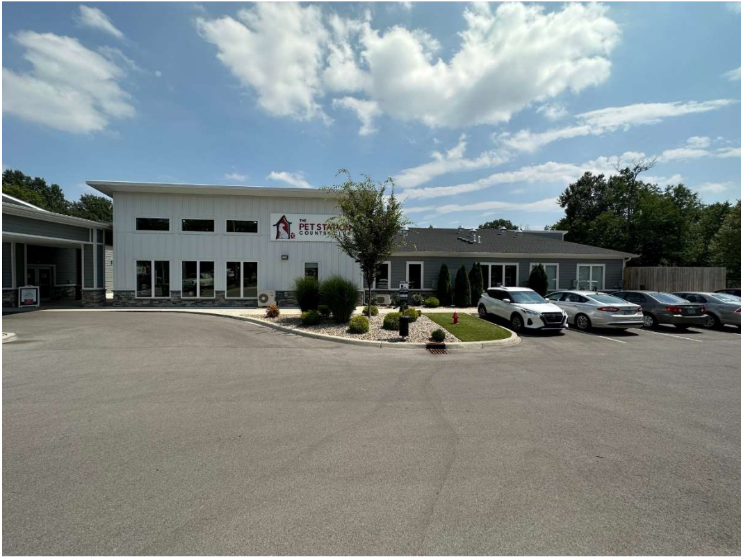
Kennel Building – Front View
