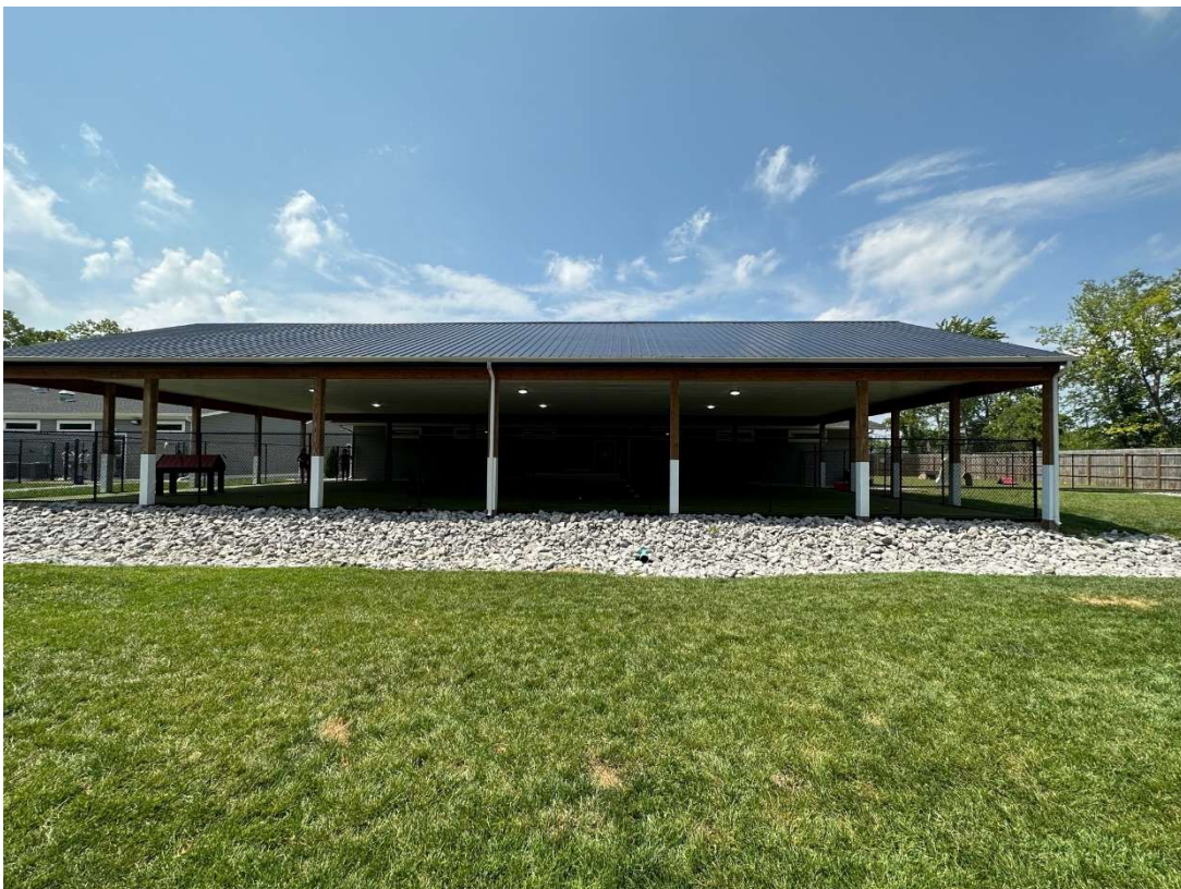
Indoor Park Building – Rear View (pavilion)
