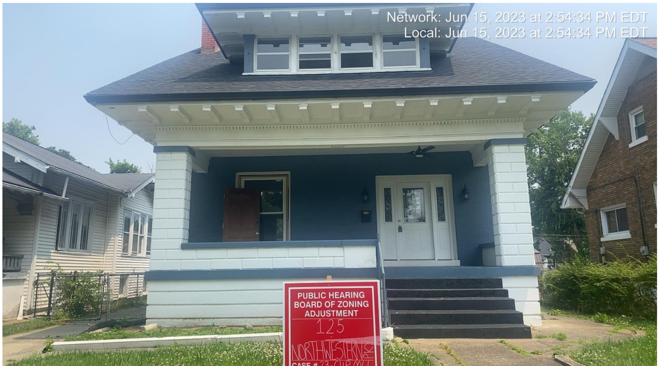
Front of subject property.
