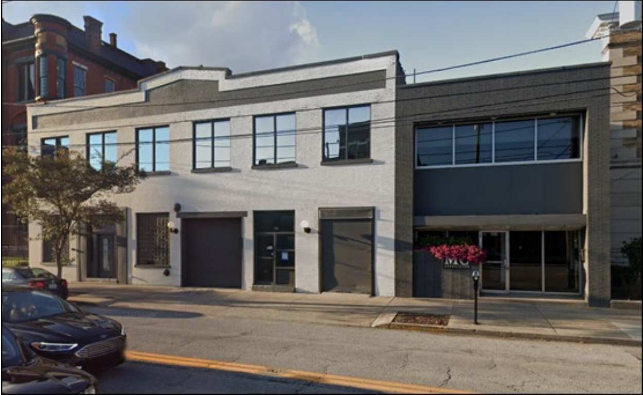
Building to be demolished, 625 E. Market - Google 2022
