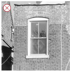
Repoint a deteriorated masonry mortar joint. Mortar bonds masonry together, permits movement, and acts as a conduit for moisture transpiration. Walls that have damaged or inappropriate mortar are at risk of freeze-thaw deterioration.
