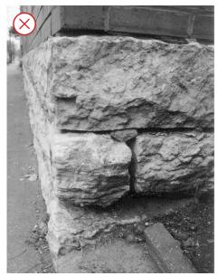
Repoint a deteriorated masonry joint. Utilize a mortar mix that is compatible with historic masonry and that will allow moisture to escape.
