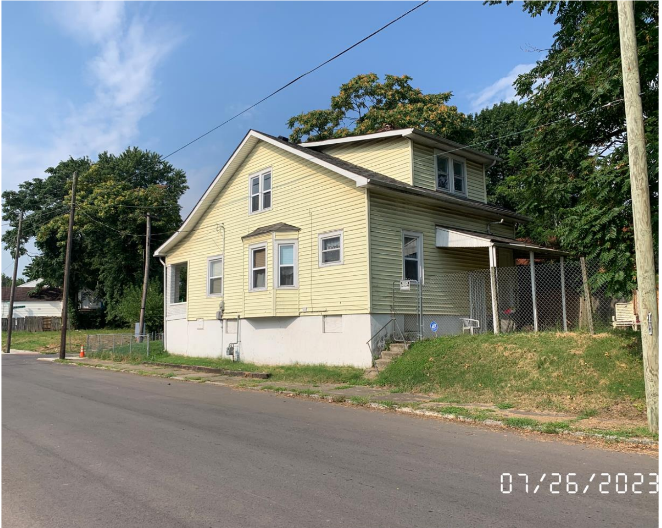
Rear of subject property.
