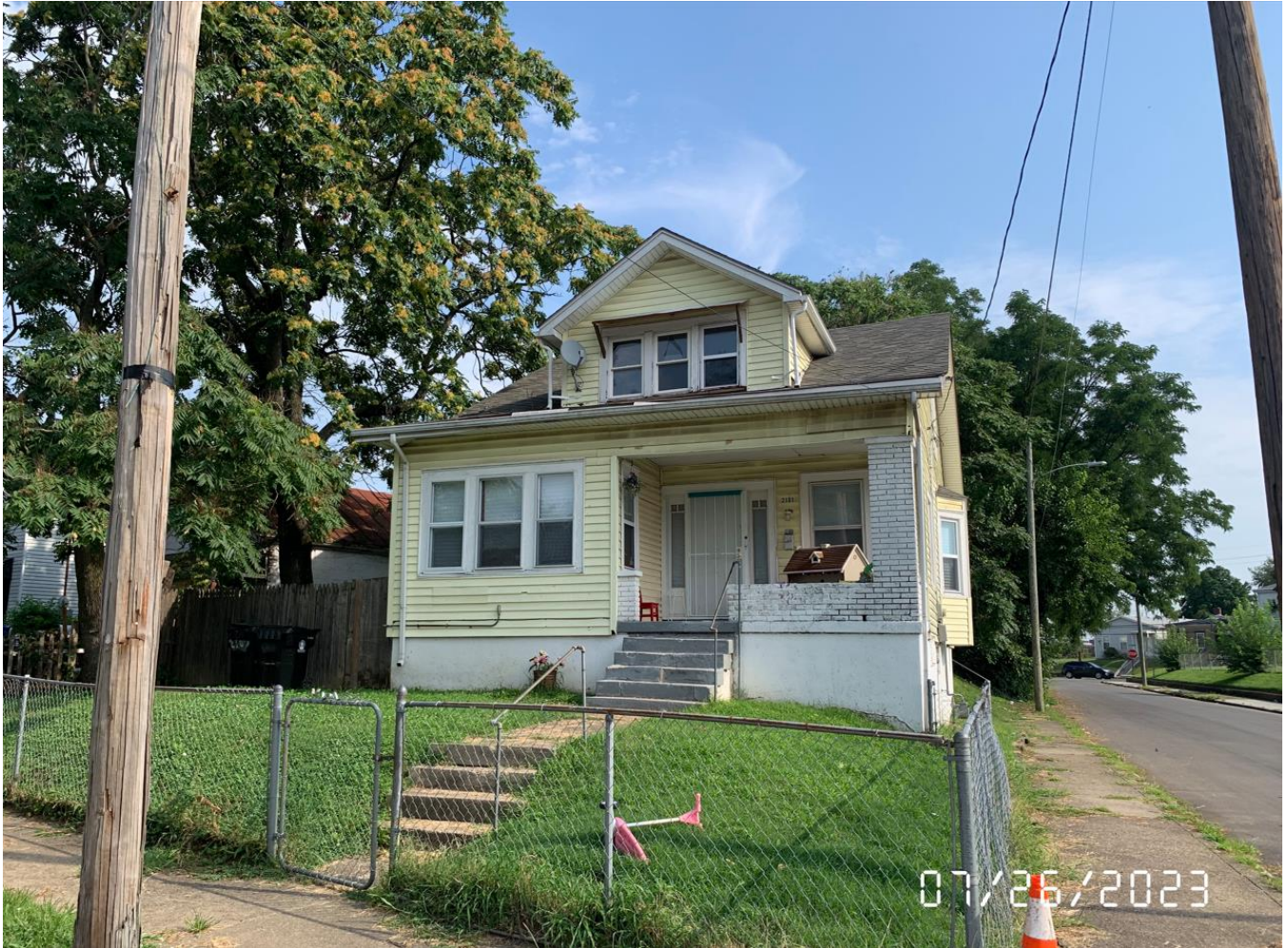
Front of subject property.
