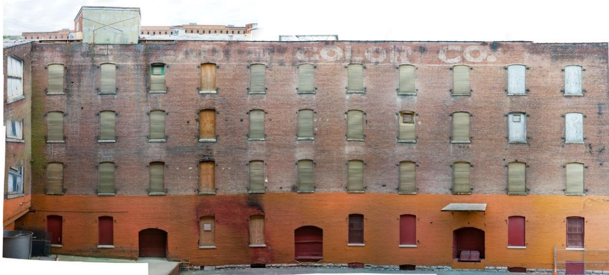
Eastern façade of ca. 1905 paint factory (Anthony Seitz/Falls City Photography)
