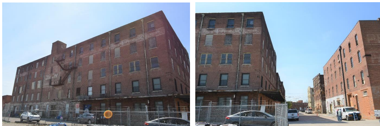
(Left) East façade of ca. 1911 warehouse addition; (Right) Facing west along Lytle Street (J. McCarron)
