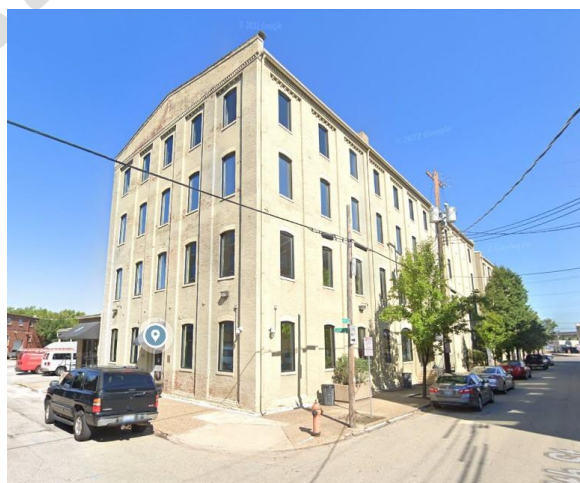
Greve, Buhrlage, and Co., ca. 1868, to the NW
