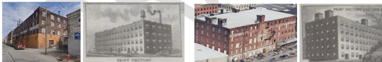
(L to R): SW corner of ca. 1905 factory; building sketch of “paint factory” from 1928 Peaslee-Gaulbert letterhead; S and E facades of ca. 1911 warehouse; building sketch of “paint factory section 2” from 1928 letterhead
