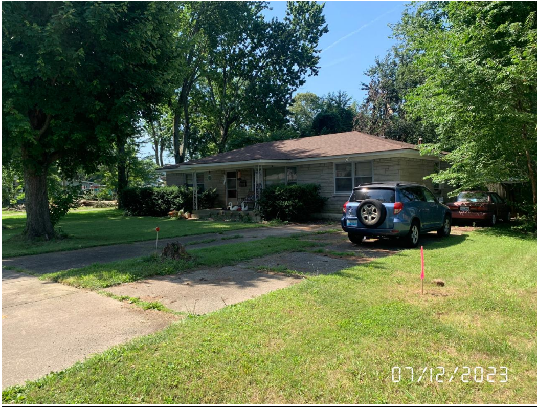
Left of subject property.
