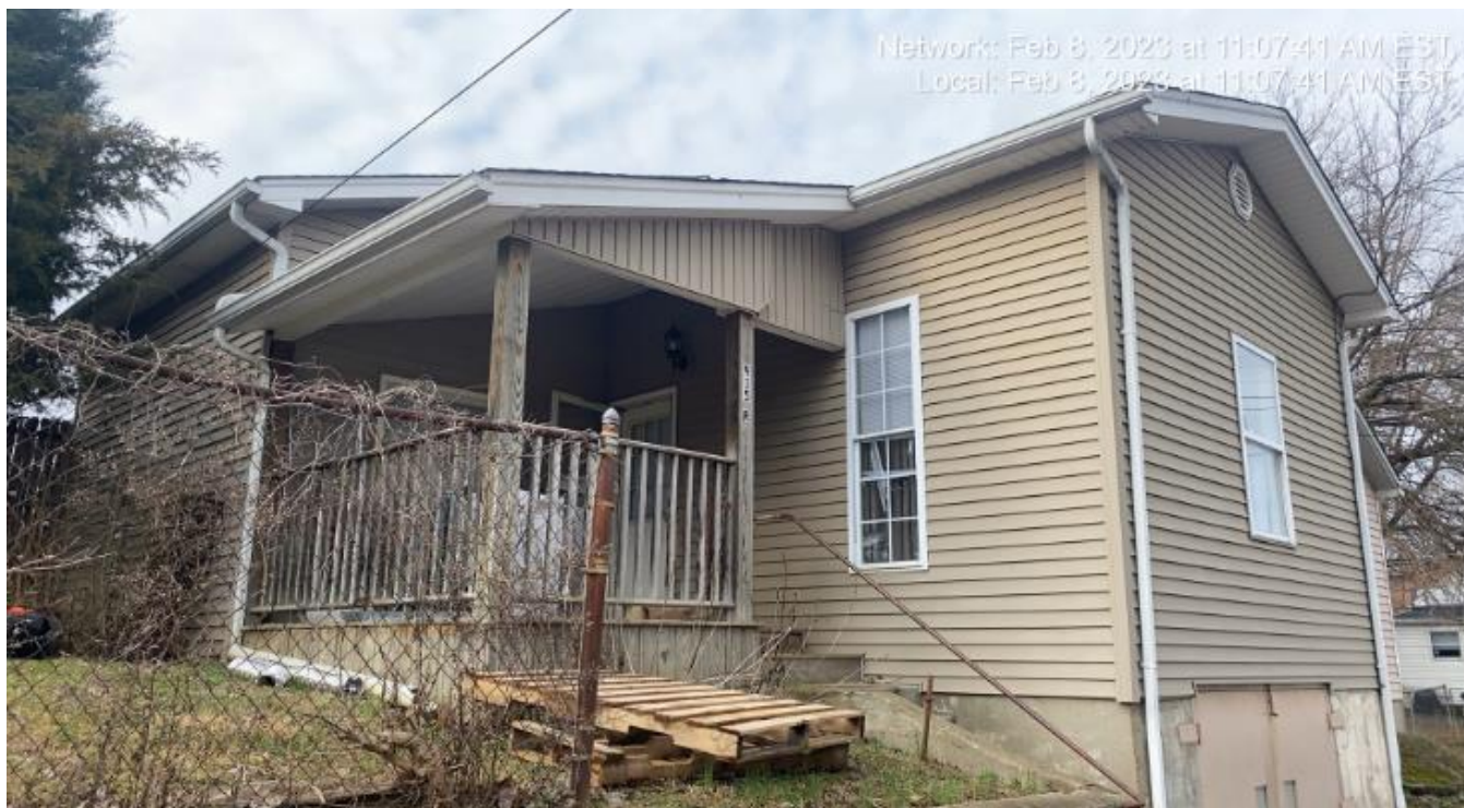
Right of the subject property.
