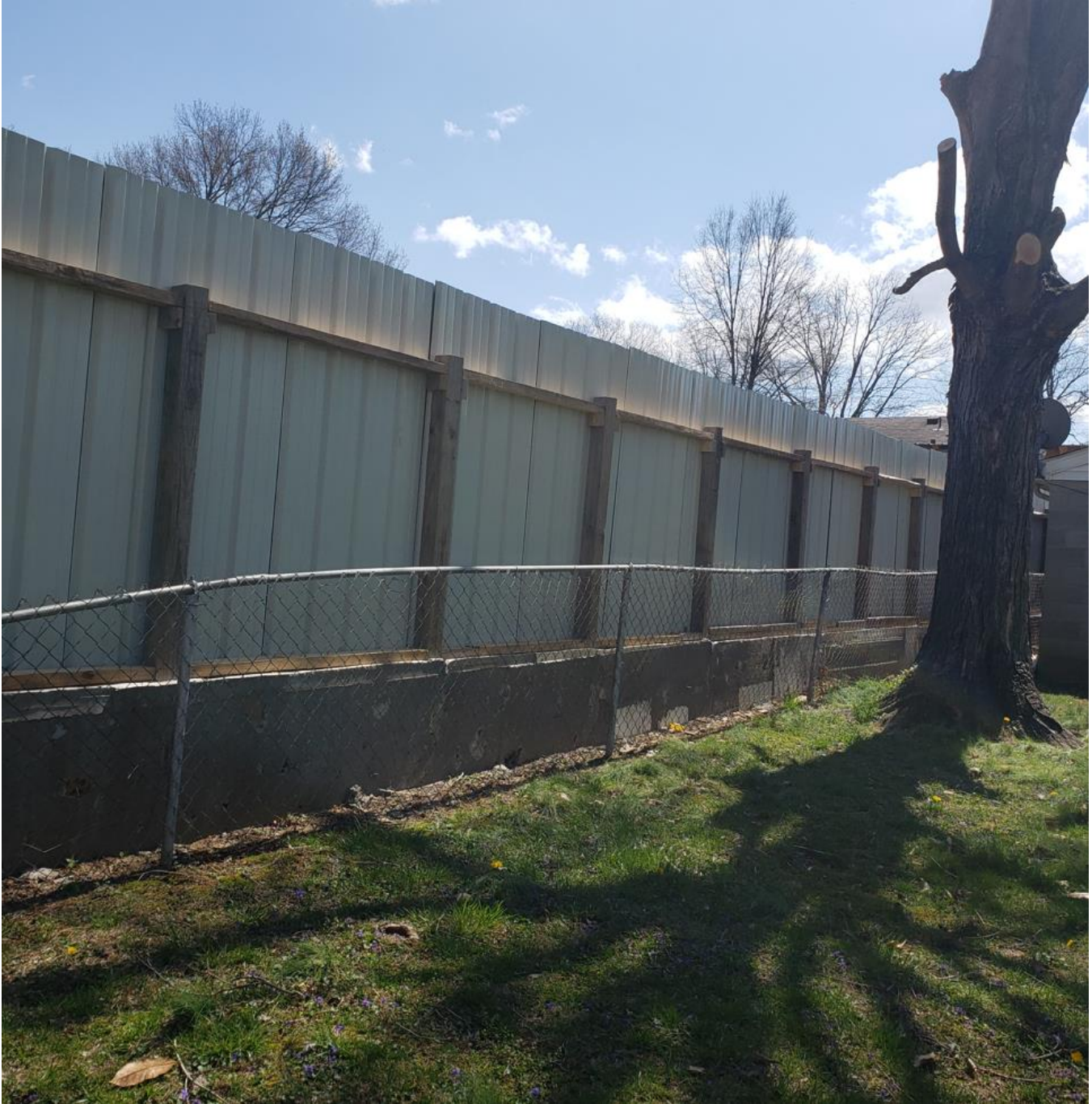
Backside of fence on rear property line.
