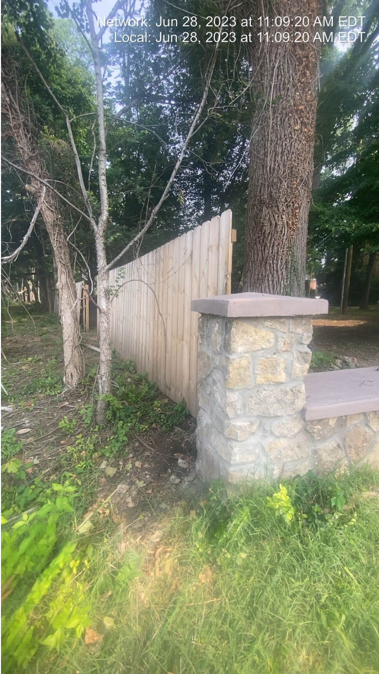
Fence in the side yard.
