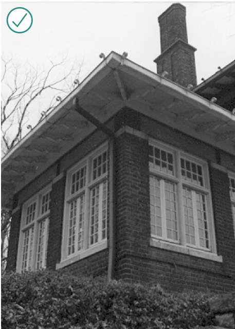
Preserve the functional and decorative features of a historic window, as well as the original window material.
