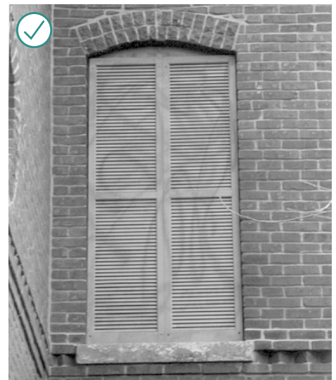
Preserve and repair existing wood shutters.
