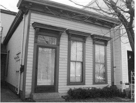
Preserve original siding and trim. Siding and trim convey architectural character and are important components of a historic building. In the top photo, three tiers of elaborate and dramatic wood trim seen in the porches, the tower, and the gable express the Queen Anne-character of this house. The bottom photo shows rectilinear wood cladding and trim that give the Italianate house a formal, geometric appearance.
