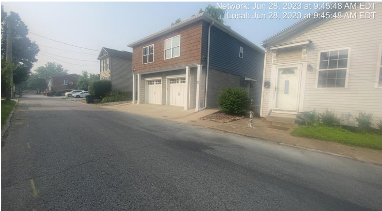
Right of the subject property.
