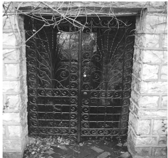
A historic metalwork door secures an Old Louisville entrance. When installing contemporary security bars, select simple designs that do not overwhelm the character of historic entrances.
