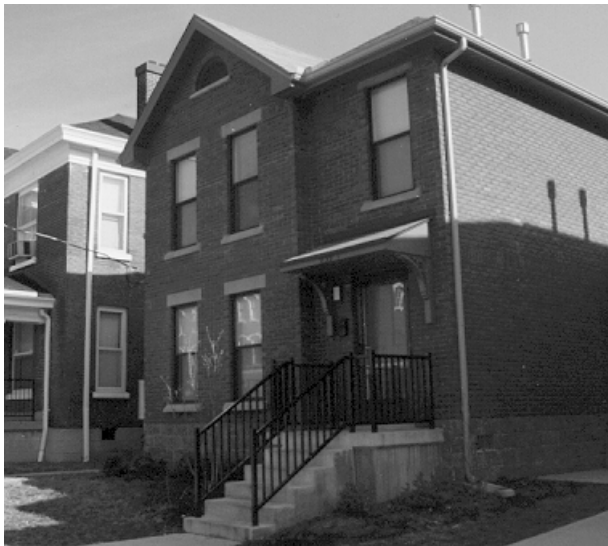
Use of a raised entry sheltered by a small, bracketed porch helps this modern building fit in with its historic neighbors. The design is simple and traditional, yet does not attempt to appear older than it really is.
