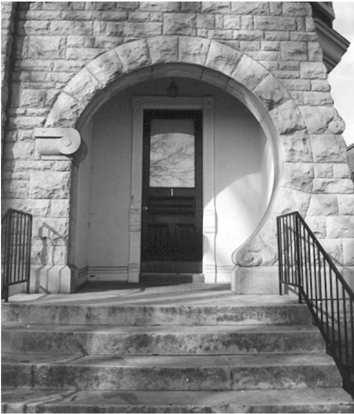
Entries help establish relationships between people and buildings. Whether imposing or inviting, the character of an entry lays the groundwork for how people relate to the structure as a whole.
