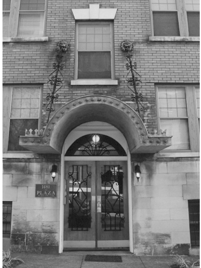
An ornate canopy with elaborate metal braces adds considerable grandeur to an Old Louisville apartment building entrance. Take a moment to imagine how different the entry would look if the canopy were removed.
